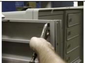
**7b. Shim spacing is needed if** the spring clip installed easily but is not securing the lock to the door adequately or if the spring clip is too tight to squeeze into place. In this case, use additional washers on the backside of the door to fill the gap so that the spring clip can secure the lock to the door using the back set of grooves.
