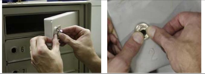
**7a. Slide the spring clip into place** through the grooves closest to the backside of the door. If needed, the pliers or the vise grip may be used to squeeze the clip into place. The lock should be tight to the door. (Note: Make sure you install the clip in the same direction it was originally installed. Also, if an AmLkr CBU, reuse the original clip.) If it is too difficult to install the clip, go to 7b.
