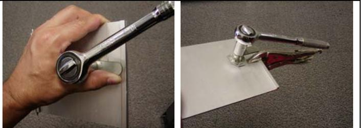
**10. Check operation of the new lock** before closing the door. If the key inserts and the plug turns without difficulty, repeat the process with door closed. If this is acceptable, then close the door and remove the key.
